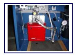
When there is a <u>modulating burner</u> (BS3/M) installed, the <u>lowest</u> possible power output must be regulated below 60kW !!! This to ensure that the CO value will not be too high. (for safety reasons).
