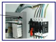
When the connection cable is connected, the main switch can be moved to position "1" and the direction of movement of the motors must be checked (to prevent damage).
